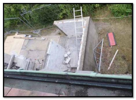
In July, work started on the Amenities Improvement Project. The first phase was demolition. This included not only the complete removal of the old porch area on the North elevation, but also removal of the existing toilet and walls dividing the toilet and kitchen area in the crypt. This whole area will now deliver a new, much larger and serviceable kitchen area.
